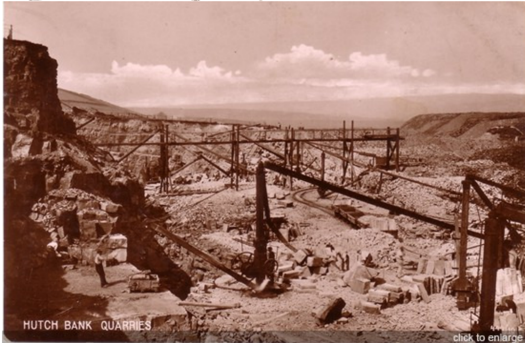
Multiple derrick cranes at Hutch Bank Quarry
