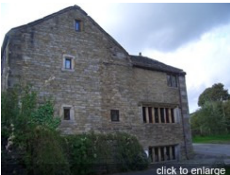
Early farm building, Waggoner Tunstead, 1632 with distinctive mullion windows, Stacksteads
