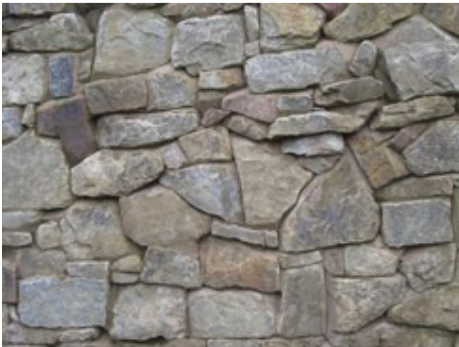
Example of random rubble walling with angular uncoursed stonework
