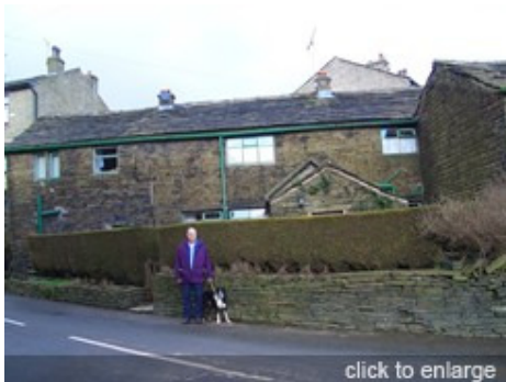
Tong End Farm showing shallow coursing in an early property, Whitworth
