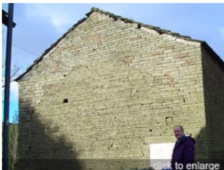
Early barn at Tong End, thicker coursed work at the top indicates a raising of roof level, Whitworth
