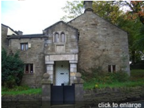
Fearn's Hall 1696, with coursed stonework and massive door porch and lintel, Stacksteads
