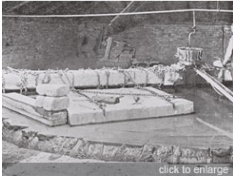
Close up of flag stone chained to beam
