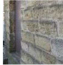
Faster building techniques needed for mills, terraced housing, bridges, and reservoirs. 'Rock-faced' pitched building stones were used and smooth polished Ashlar stone on the most expensive buildings.
