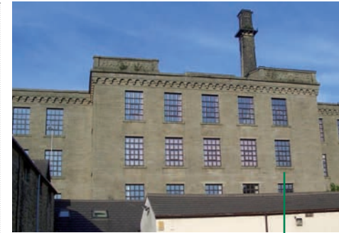
3 ) High quality masonry from Horncliffe quarry
