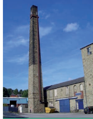
13) Atherton Holme Mill chimney, one of the few surviving chimneys in Bacup
