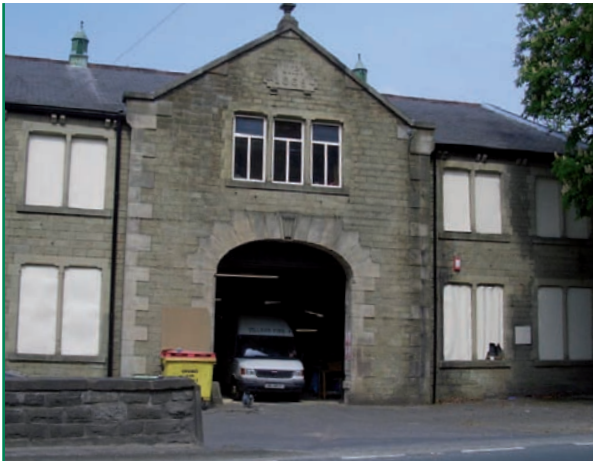
15) Punch faced masonry and overall symmetry
